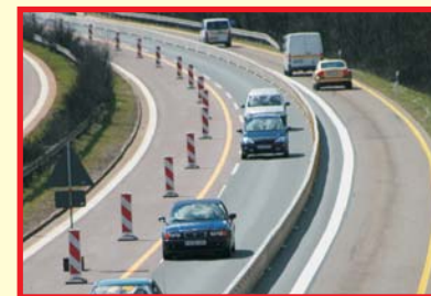
Lane switches and transition zones are no problem with ProTec for safe, clearly recognizable traffic control.
