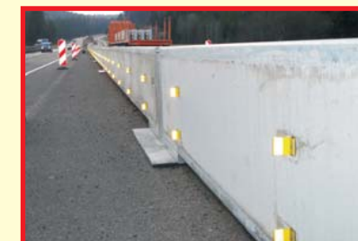
The retractable reflectors are fitted into the concrete in such a way that they recede when touched and are preserved even when a vehicle touches the barrier.
