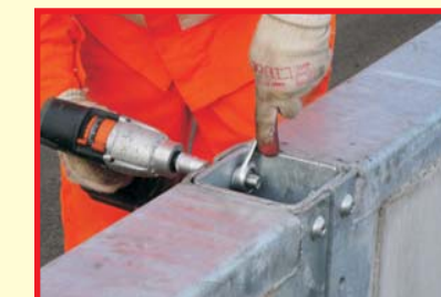
Fast installation: one stand is always fitted to every element. All it takes is to screw in two bolts every 10 m.
