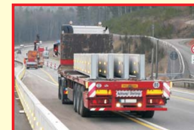
Up to 80 m of ProTec 160 can be loaded on a truck and installed directly from the vehicle.
